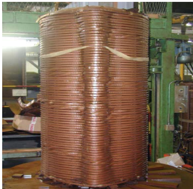
Fig. 5: Deformation of winding due to short circuit.
